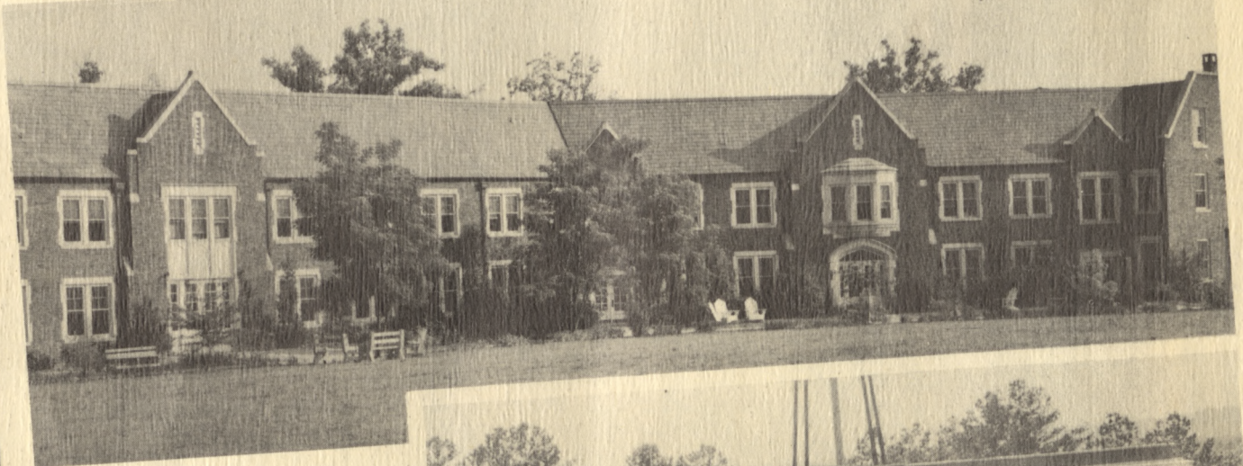
DAUGETTE HALL DORMITORY
