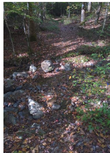
Figure 39. Overflow erosion near area 3 (Photo Credit: Allie Field, Jacksonville State University Trails Science Institute)
