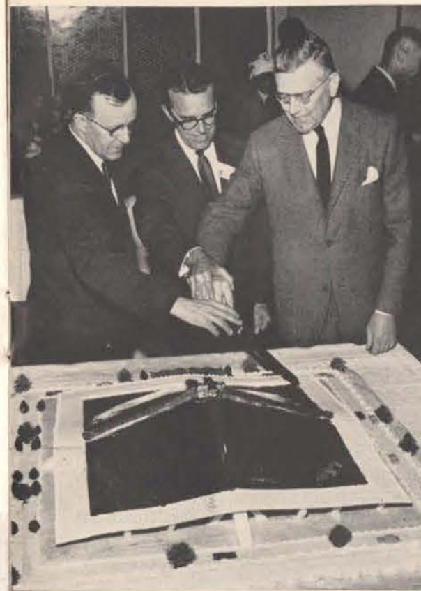
During ground-breaking ceremonies for the Century 21 Coliseum, three notables join in cutting a cake modelled after the structure. They are: speaker of the day Dr. John P. Hagen, of the National Aeronautics and Space Administration; Seattle Rotarian Edward E. Carlson, chairman of the board of Century 21; and Paul Thiry, primary architect of the building—which has no interior supports.
