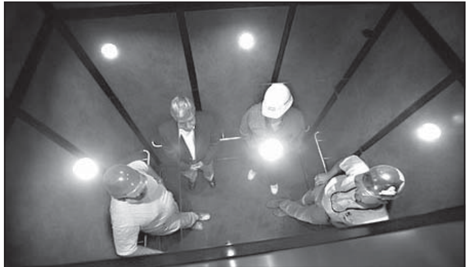
Above: JSU's Miller Parnell (hatless), along with contractors, takes a test ride in the first of the newly installed elevators. The photo was shot in the reflection in the cab's mirrored ceiling. Below, left: The elevator shaft-- a study of perspective. Which way is up? Below, right: A ThyssenKrupp employee works toward putting the wheels in motion. (Steve Latham Photos)
